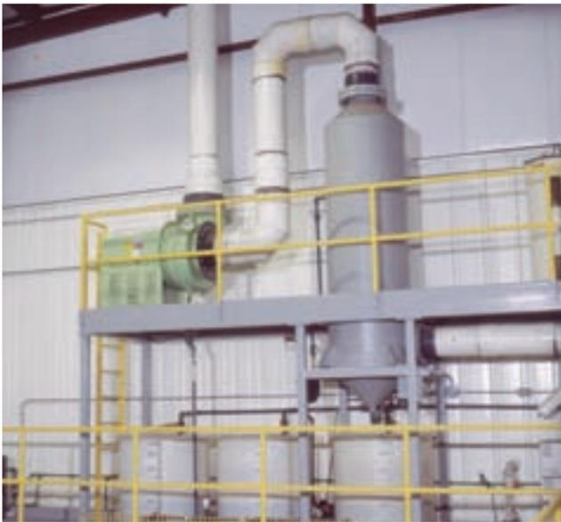
**Gas Scrubber Removes Hazardous Vapors** — An Impinjet® gas scrubber has been employed by a major producer of industrial chemicals to remove hazardous (noxious) vapors. The scrubber vents both bottle filling and dry bulk filling areas at the company, which produces hydrochloric, sulfuric and nitric acid as well as formaldehyde and ammonia.
